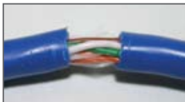
Bend cable, remove jacket
